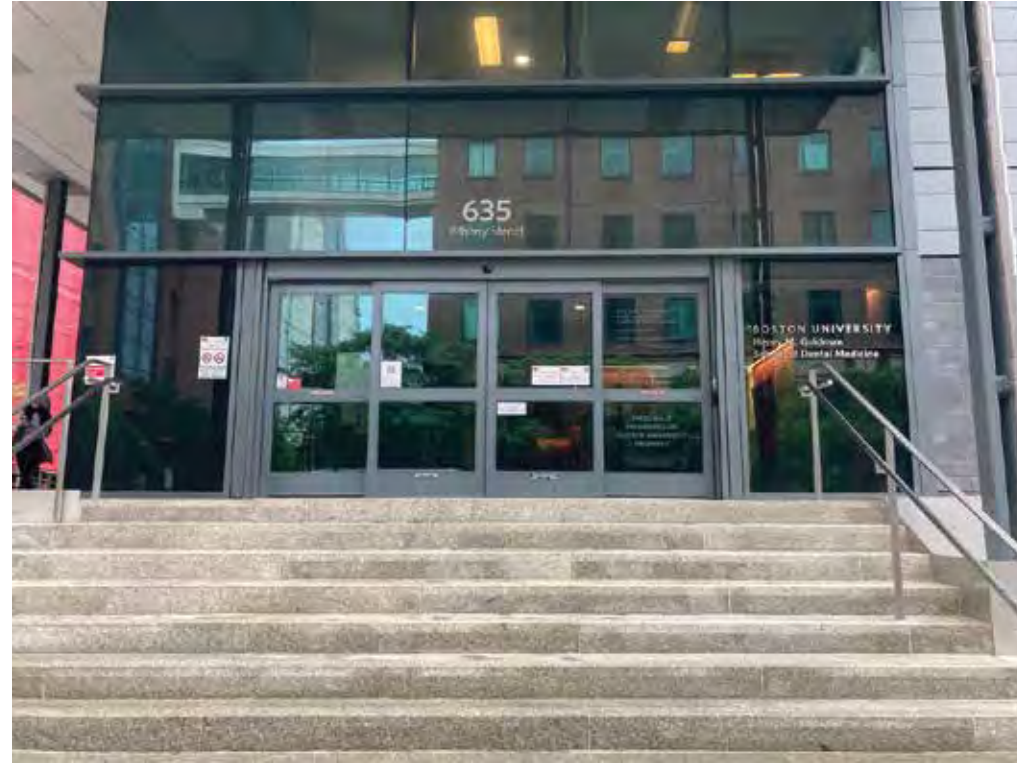
Location 16: Building Identification
