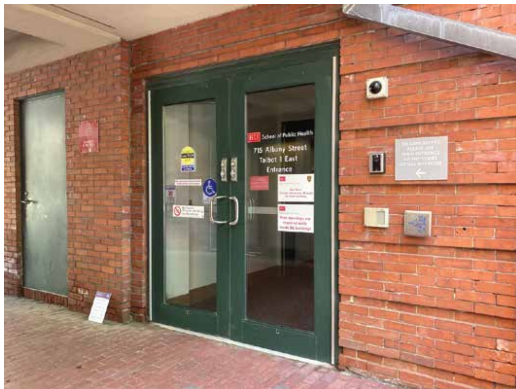
Location 13: Building Identification & Entry Information
