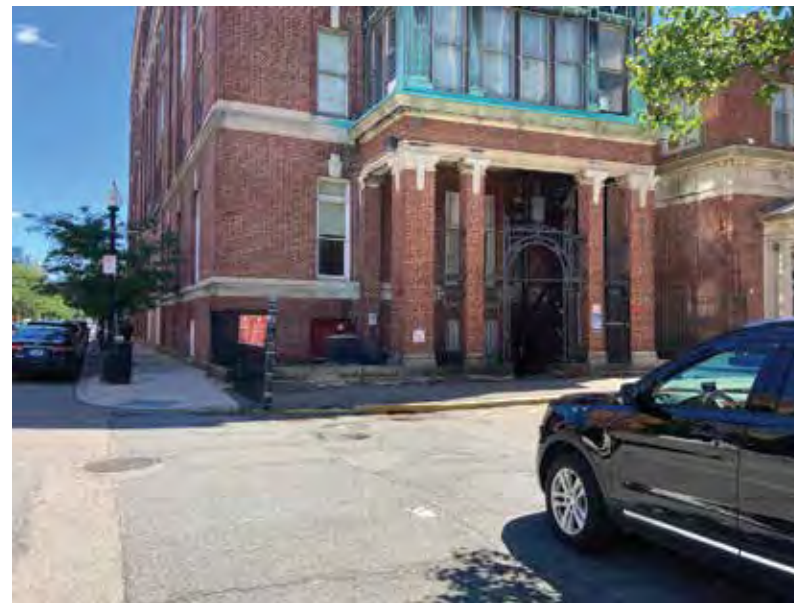
Location 36: Building Identification
