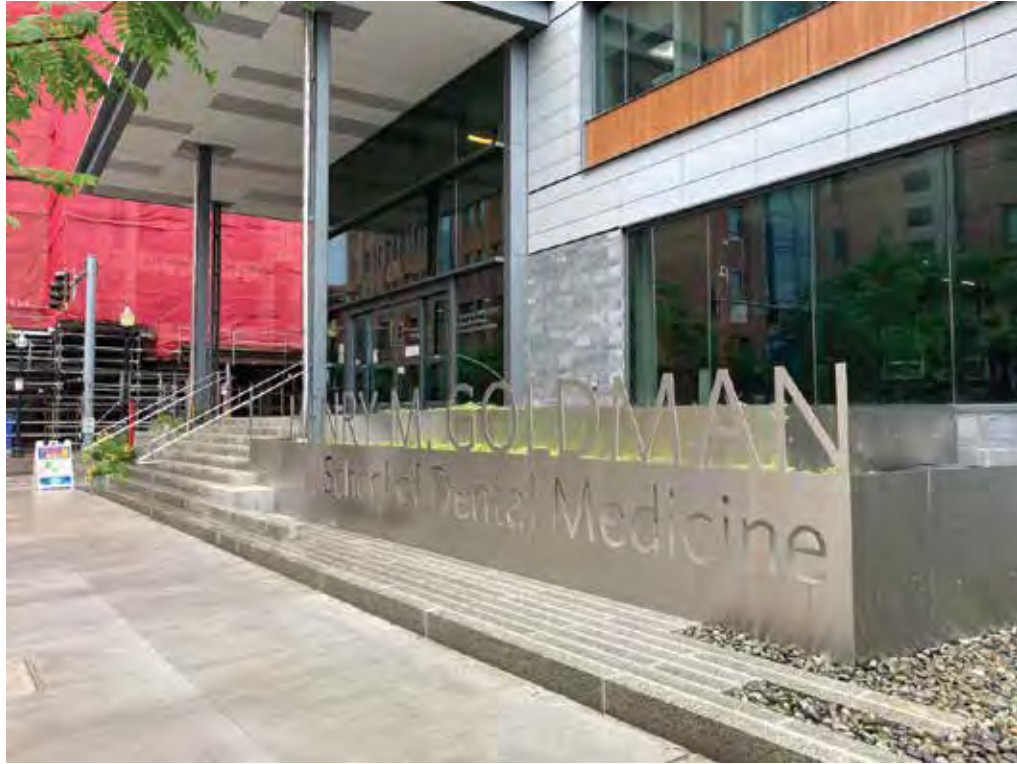
Location 15: Building Identification
