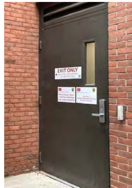
Location 29: Building Identification & Entry Information
