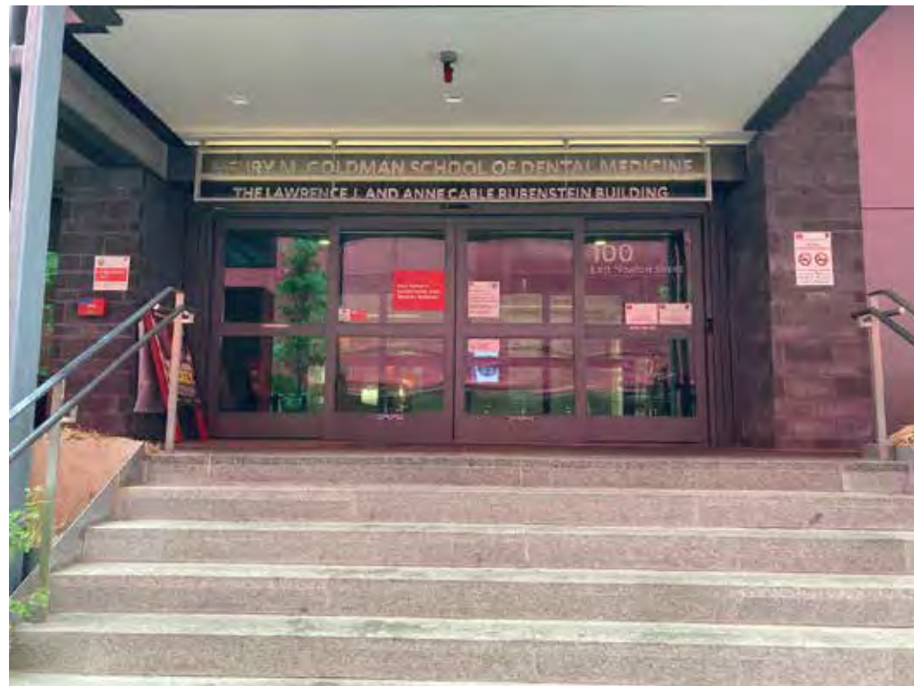
Location 18: Building Identification
