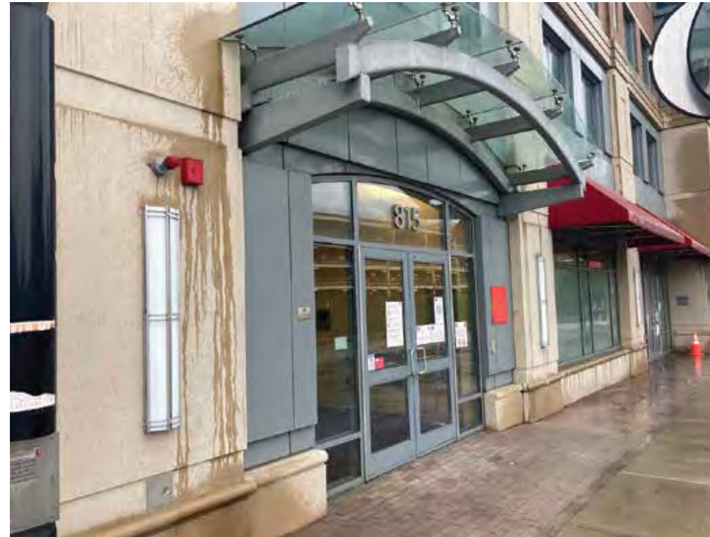
Location 40: Building Identification
