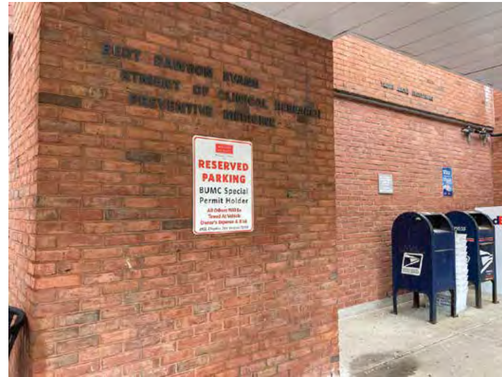
Location 28: Building Identification
